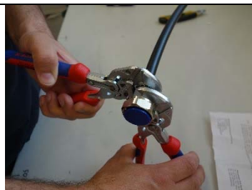
20) Tighten connector head and back nut with wrenches until stop. ( Recommended torque: 15 Nm)
